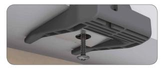
3. Keeping the tool in place, either drill a pilot hole through the centre of the holes on the bracket, or - if fitting to a suitable substrate - directly drive a screw up into the recess until tight. Ensure the tool stays flat and square against the recess while doing this. Once the screw is tight, the tool can be pulled out of the bracket.
