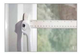
1. Ensure there is at least a 25mm clearance from the edge of the visable glass to any handles or air vents.
